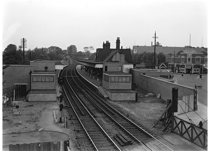
Leytonstone station on 15 July 1942. Then owned by the London & North Eastern Railway, this wartime view shows the station as a mixture of old and new. The electric conductor rails are in place for the anticipated Central Line tube trains, but they wouldn't appear for a further five years.
